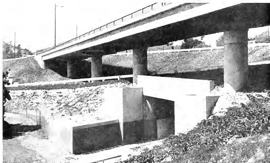
Looking northwesterly showing in foreground Ivor Street underpass with Cahuenga Boulevard eastbound on-ramp over it and with the Franklin Avenue off-ramp above. This constitutes a three-level interchange.
